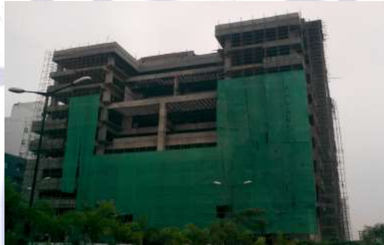
Building warping by geo textile fabric
