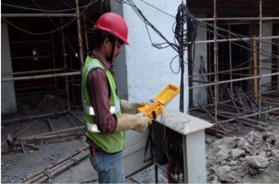
Utalika- Sensitivity test of Residual Current Circuit Breakers
