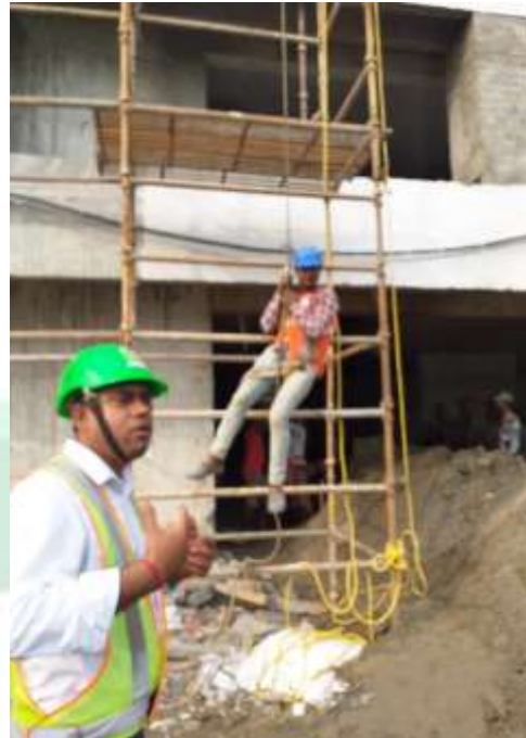
Utalika- Live demo on Use of Fall arrestor
