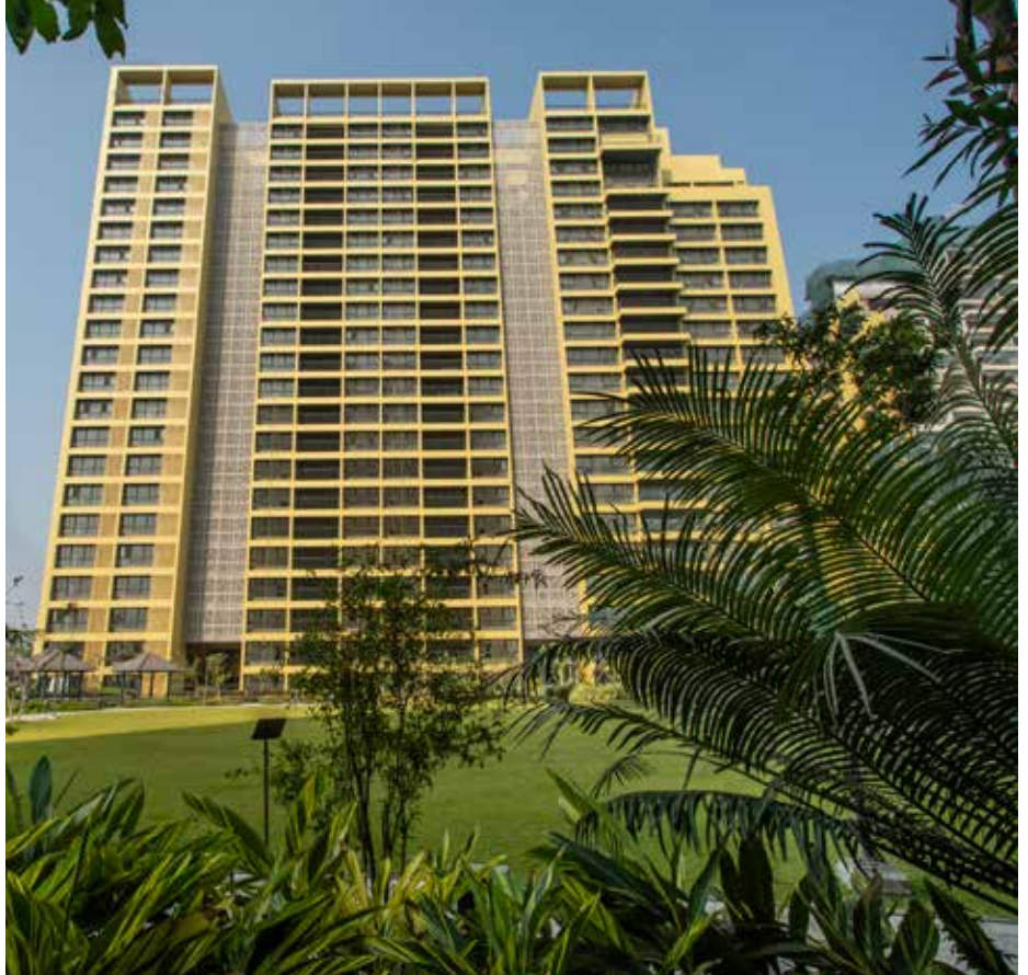
A panoramic view of the Prathama tower
