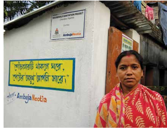
In sync with Swacch Bharat Abhiyan, household toilets were constructed in and around Rajarhat
