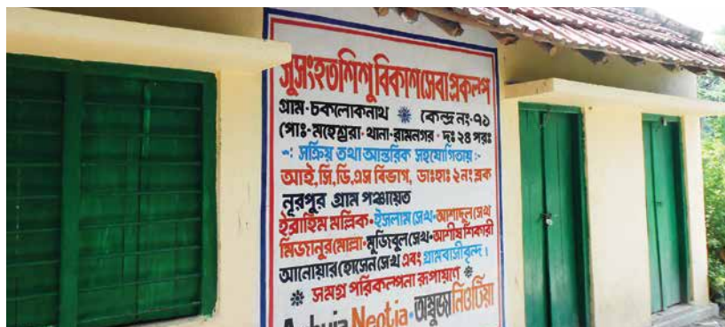
We have helped to build an ICDS school at Raichak to ensure education for boys and girls in the local villages
